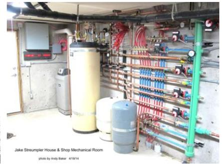
Jake Struempler is a mechanical contractor and innovator who has successfully completed a very ambitious and innovative solar thermal collection/storage/distribution system on his large shop building/hangar. Below the floor he has excavated a 36ft x 36ft x 8 ft deep pit and filled it with wet sandy gravel to make an earth heat storage battery. The battery is lined with 4" blueboard + radiant barrier to keep heat from escaping to the surrounding ground.
