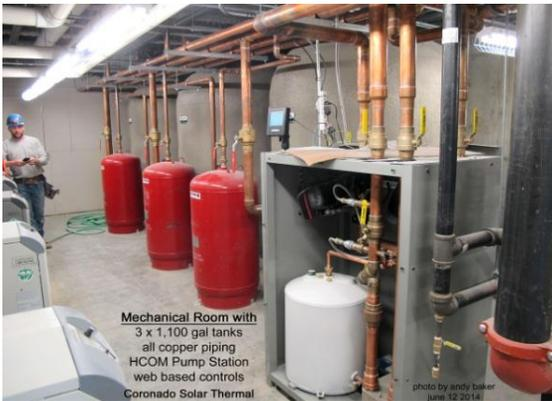
Mechanical Room with 3 x 1,100 gal tanks all copper piping HCOM Pump Station web based controls Coronado Solar Thermal
